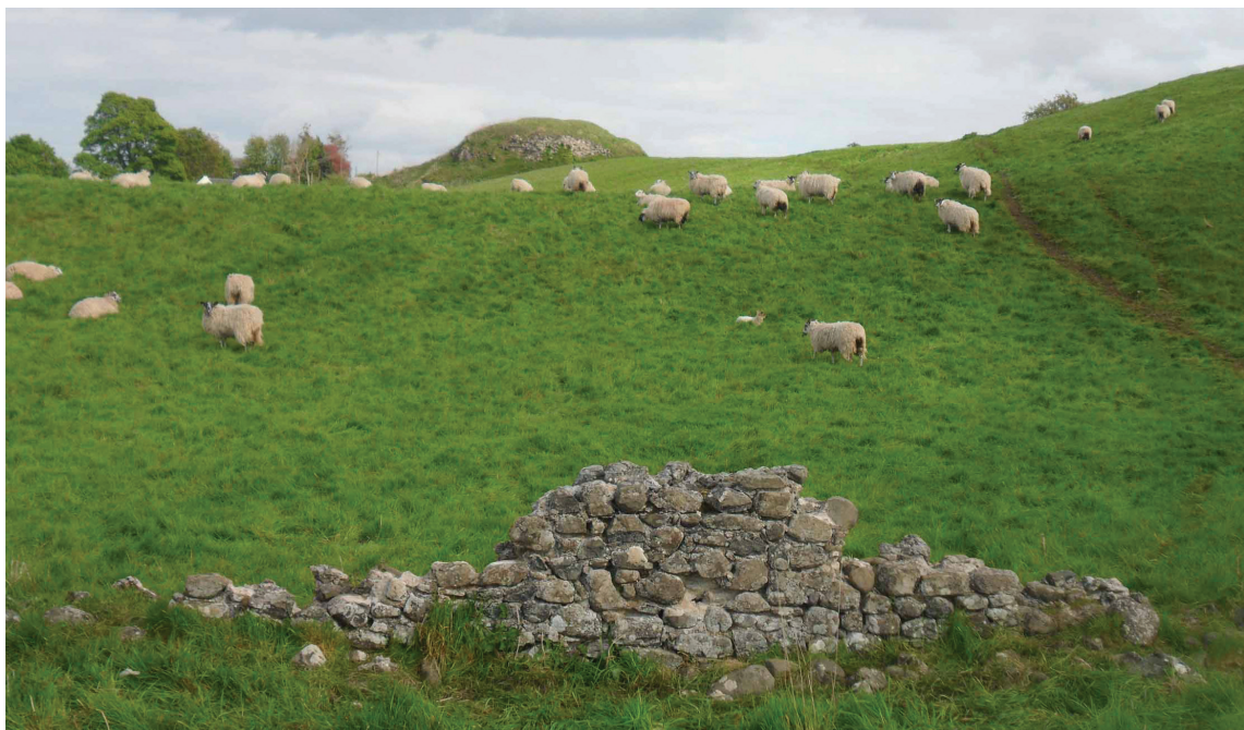
View eastwards of part of St. Giles's cemetery wall with the castle mound to the rear
